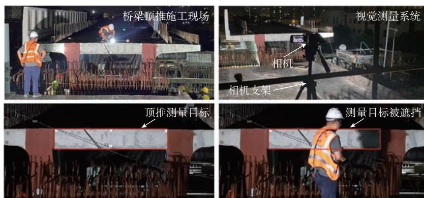
图 24 桥梁顶推施工现场中测量目标被遮挡 [131] Fig.24 Obstructed measurement target in bridge launching construction site [131]
