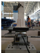
图12 某型机后机身装配现场 Fig.12 Assembly scene for the rear fuselage
