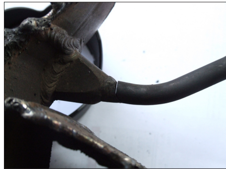
图1 进油管外观及开裂部位 Fig.1 Appearance and crack position of vitta
